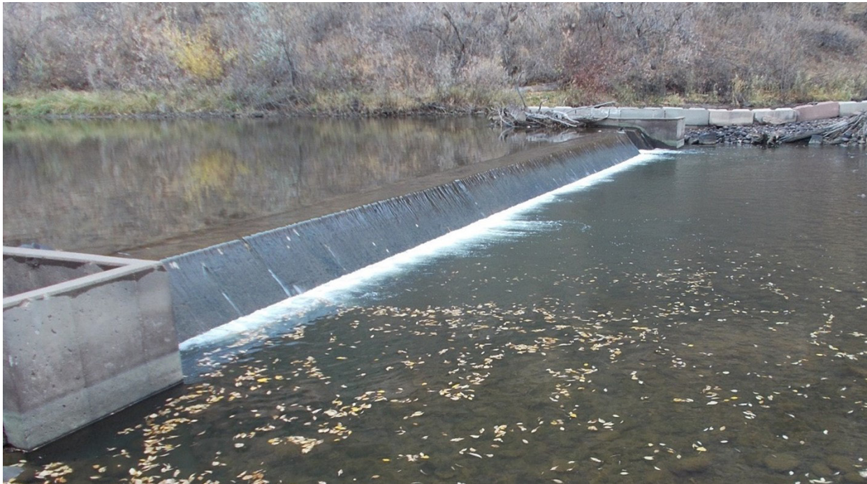
Figure 1: Jackson Ditch Diversion Dam, Cache la Poudre River near Ft. Collins, Colorado. August 30, 2018. Photographed by Karl Kingery of Wright Water Engineers, Inc.
