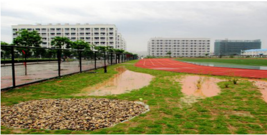
Figure 3. Infiltration Area and Swales in Foshan, China Source: Shaw L. Yu
