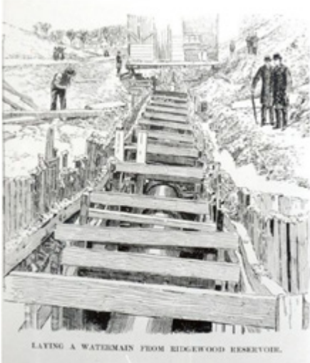
Image 1: Depiction of water mains being laid from the Ridgewood Reservoir, 1867
